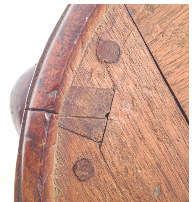
Dovetail and peg construction detail on seat frame of Logan Queen Anne chairs.
